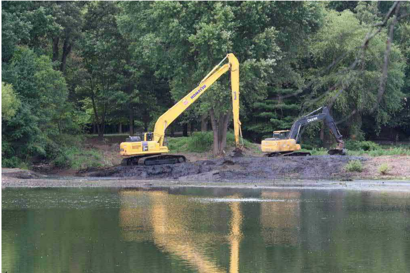
Figure 7: Long Reach Backhoe at Work
