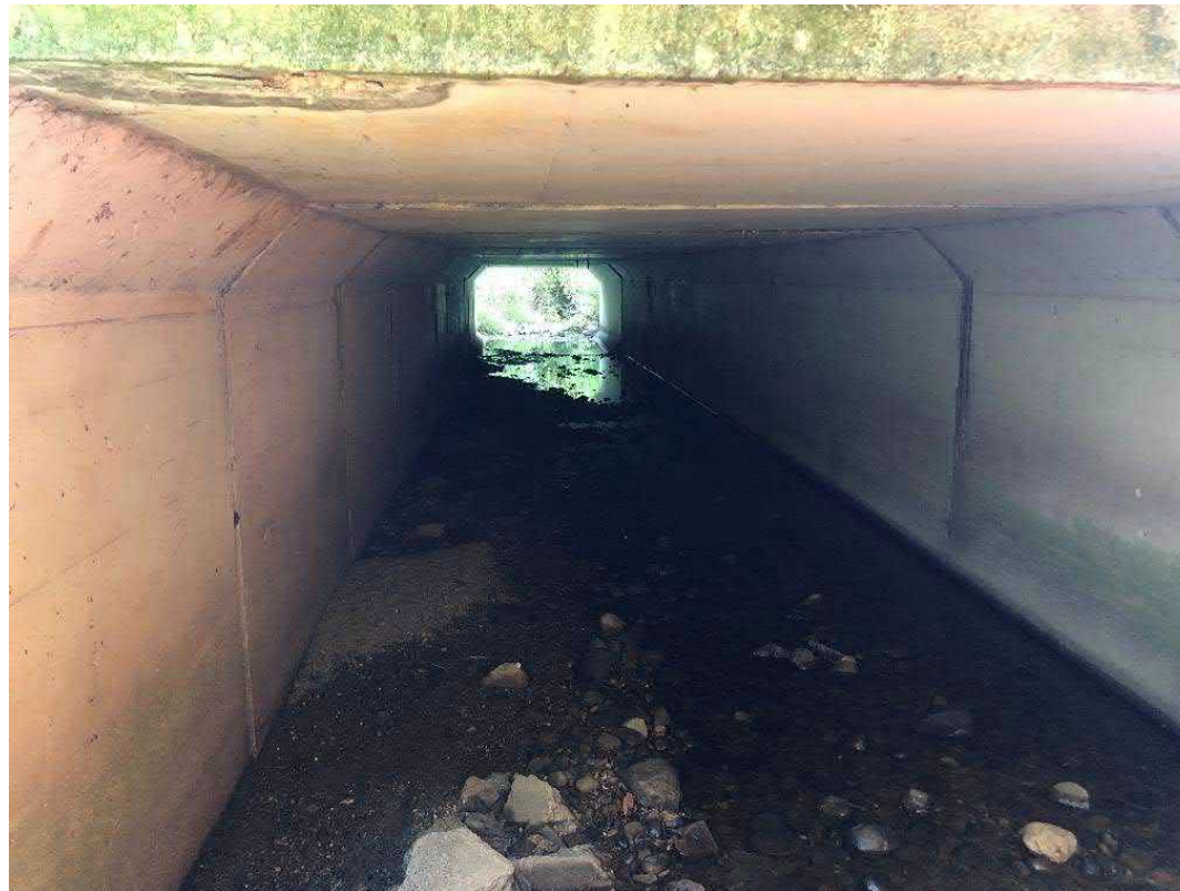
Culvert under Fulton Dr.
