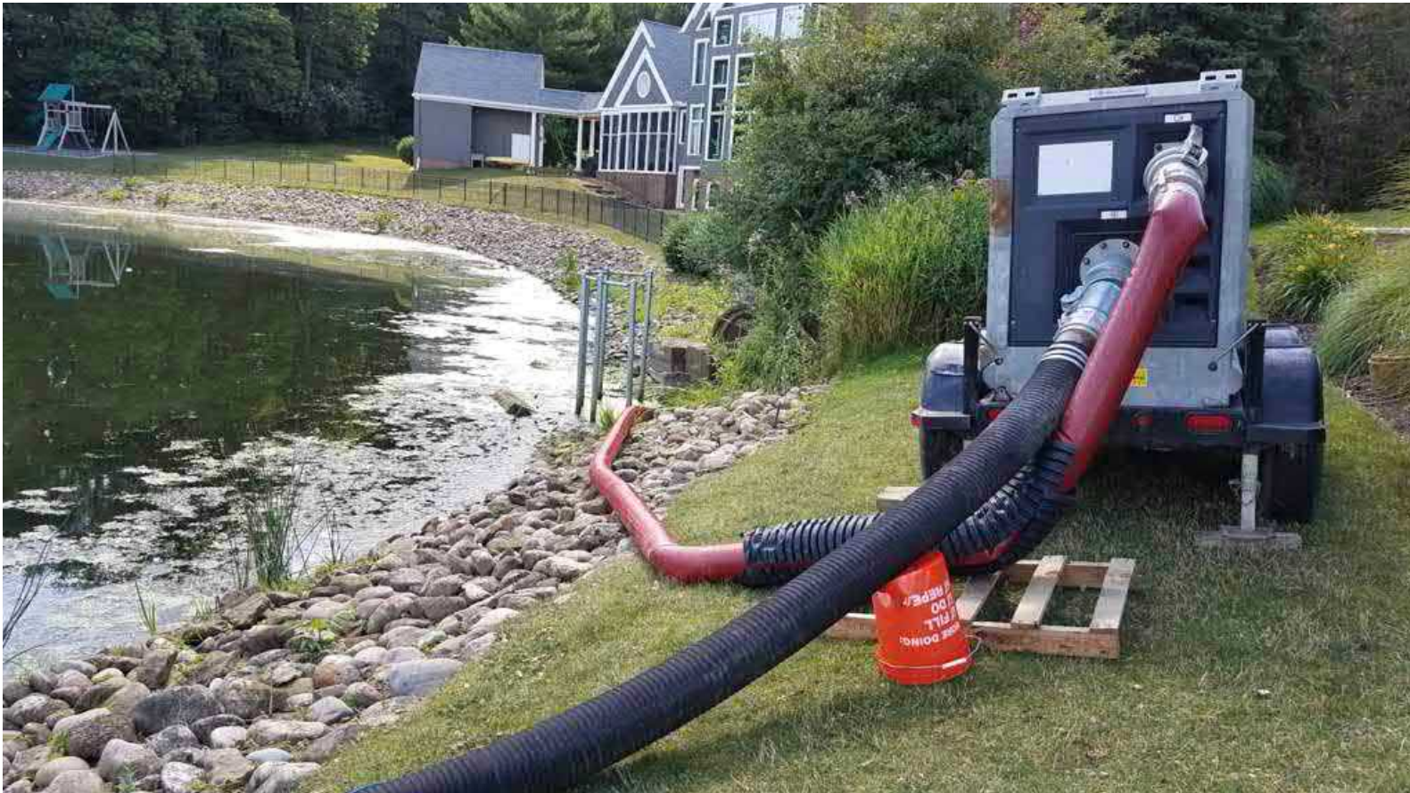
Figure 2: Diesel Driven Water Pump
