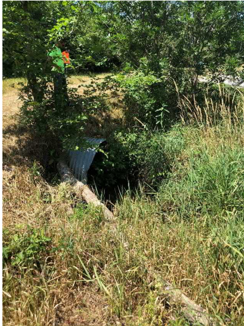
Large corrugated pipe culvert
