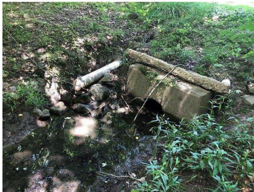
Partially buried culvert
