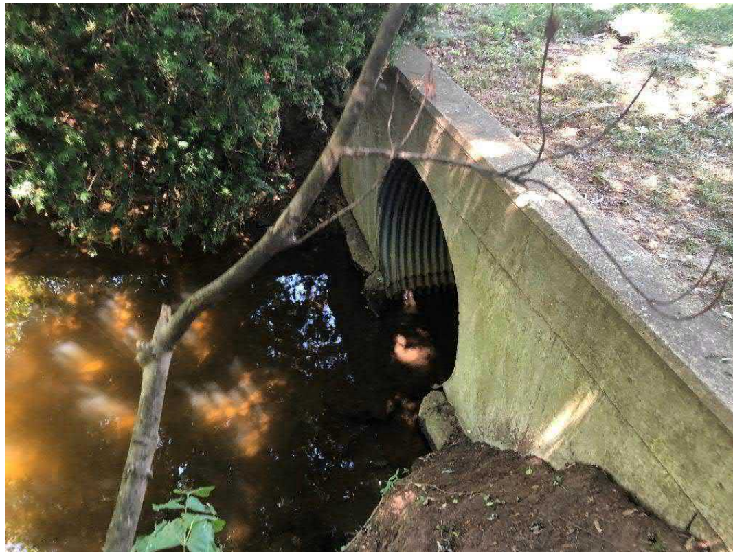
Culvert at Roger Ave
