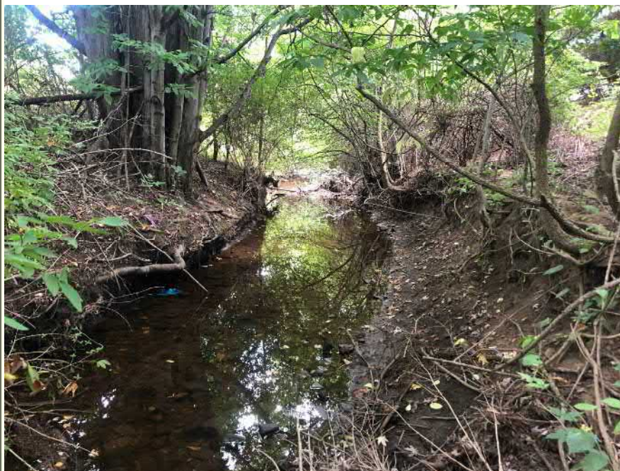
Looking Downstream. Toe and Bank Erosion
