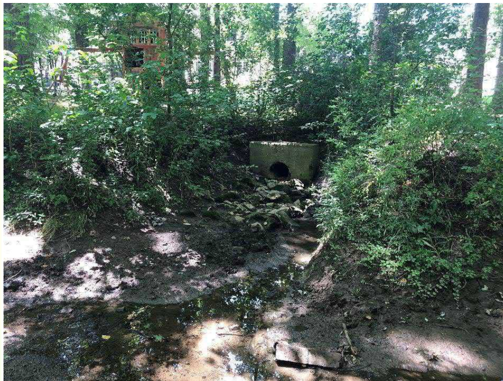
Stormwater outlet to stream
