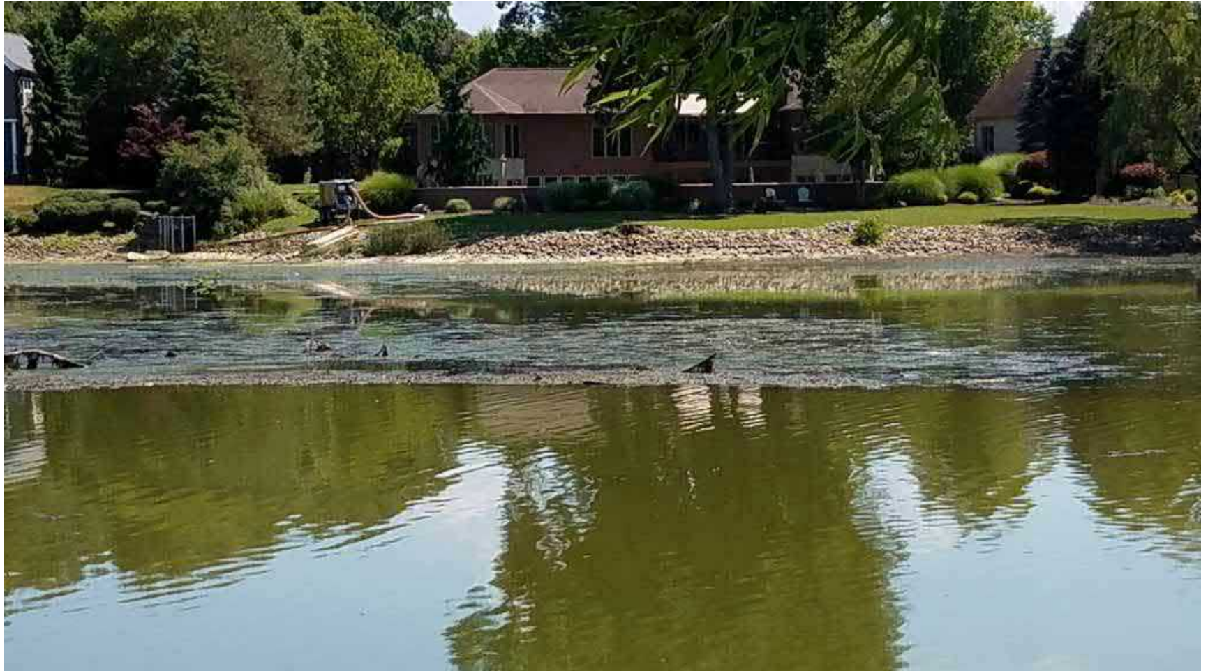
Figure 5: Sandbar South Shoreline Outlet Pipe
