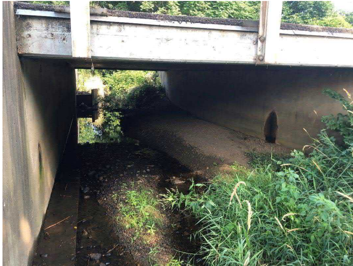
Bridge culvert at Wales Ave
