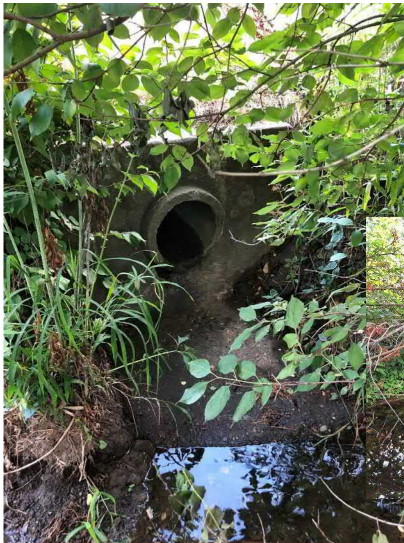
Stormwater outlets to stream
