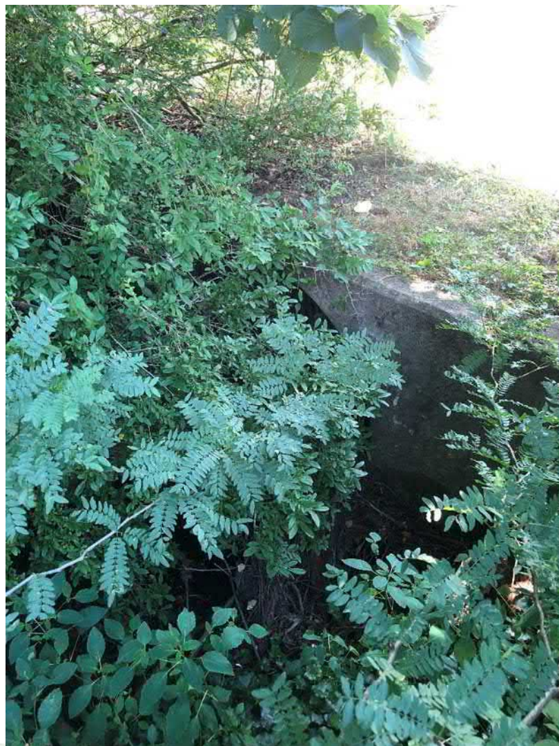
Culvert at Dale Ave
