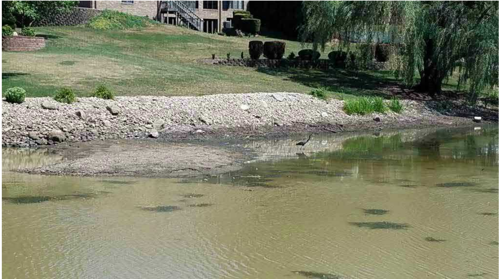
Figure 3: Woods/Meadows Inlet Pipe Area
